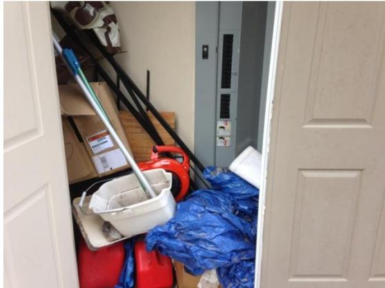
The electric panel access is blocked by lawn equipment and gas containers. This is a fire and safety violation.
