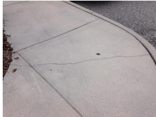
The cracking is minor and difficult to see in the wall finish. In my opinion, the cracks above are NOT indicative of structural failure, nor differential settlement.
